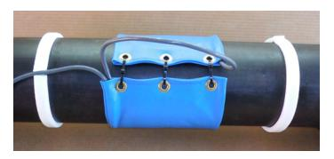
Install treatment pads opposing each other using 6 cable ties provided. Mark the pipe and install weather stripping.
